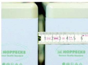
Fig. 5-14: 10 mm clearance between the batteries
