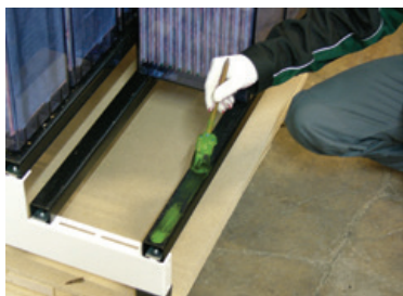
Fig. 5-13: Greased support profiles
