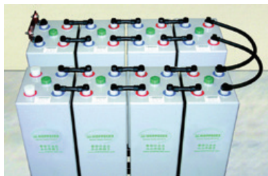
Fig. 5-15: Using row connectors and step connectors
